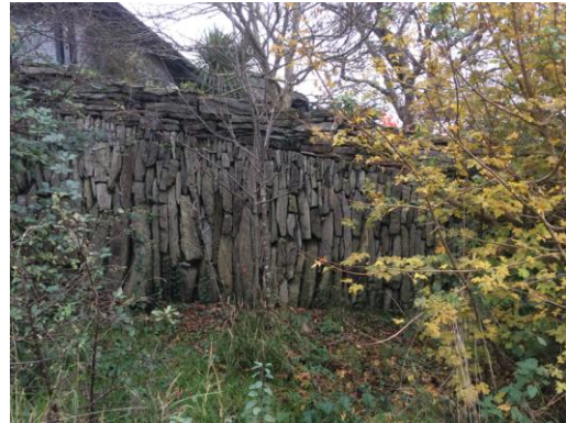
Figure 120: Distinctive stone wall pattern, Restronguet Point.
