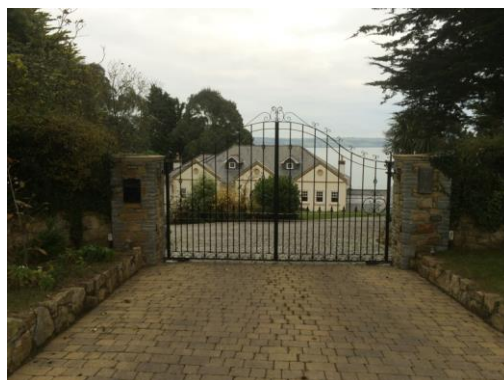
Figure 109: Open fretwork gates allow public views to the water.
