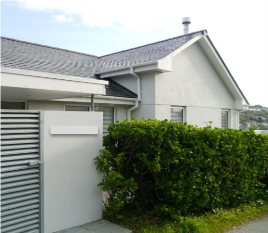
Figure 12: Modern bungalow, Point.
