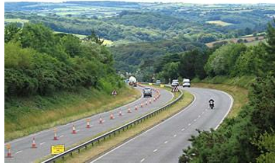
Figure 20: A39 Devoran bypass.
