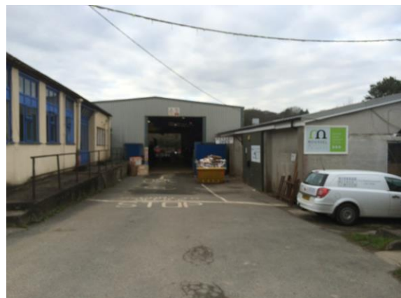
Figure 13: Devoran Metals, Greenbank Road, Devoran.
