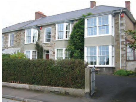
Nos. 4 and 6 Devoran Lane
