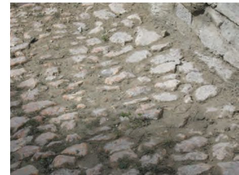
Cobbled pavements in Carlew Terrace and Quay Road
